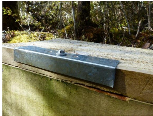
Galv bracket to protect timber around top screw
