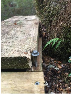
Kea damage around top screw
